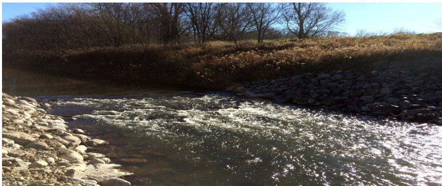
Water flowed over one of 18 rock riffles constructed within a 5-mile stretch of the Sand Hill River.
