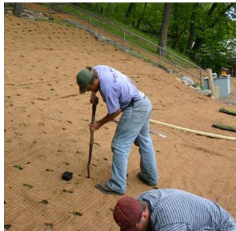
Figure 5.93 Planting containerized plants, Photo by Prairie Restorations, Inc.
