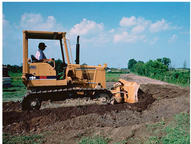
Figure 5.62 Sediment Removal
