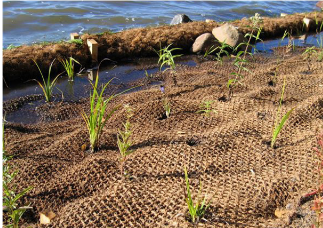
Figure 5.67 Shoreline Planting with Erosion Control, Photo by Prairie Restorations Inc.
