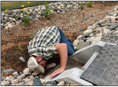
Left: Andy Arens, Itasca SWCD manager and water plan coordinator, checks on the rain gardens and sediment traps, which reduce how much sediment enters Trout Lake. Middle: Bottlebrush is among the species planted. Right: Vandyke Elementary School overlooks Trout Lake in Coleraine. Teachers worked fourth-graders’ rain garden planting into lesson plans. On the day of the planting, Earth science lessons included how communities’ water use can affect water supply and quality. Photo Credits: Ann Wessel, BWSR
