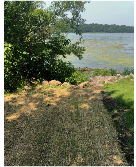
AFTER: The completed project, seen here on July 21, 2021, incorporated new tile and a regraded slope covered by erosion control fabric made of jute. It will keep an estimated 2.1 tons of sediment and 2.1 pounds of phosphorus out of Circle Lake each year.
