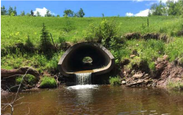
Photos: example of poor stream connectivity due to a perched culvert (l), and a completed stream reconnect project with improved stream connectivity and streambank habitat (r).
