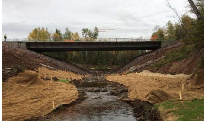
Photos: example of poor stream connectivity due to a perched culvert (l), and a completed stream reconnect project with improved stream connectivity and streambank habitat (r).
