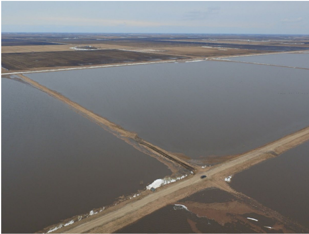
Figure 11. North Ottawa impoundment in the Bois de Sioux watershed district: 1,920 acres (3.5 sections) which holds 18,000 acre-feet of runoff.
