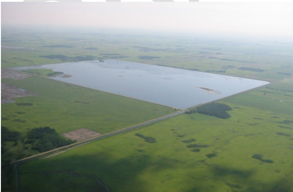
Figure 10. Off-channel Euclid East impoundment, Red Lake Watershed District. Provides detention of 2,443 ac-feet of runoff
