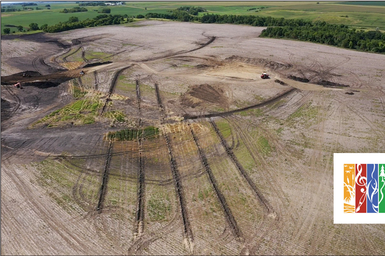
An aerial view shows the trenches where a crew from the excavating contractor Hormann Works LLC of Dumont installed tile as part of the project involving eight water and sediment control basins in Henrichs' field.
