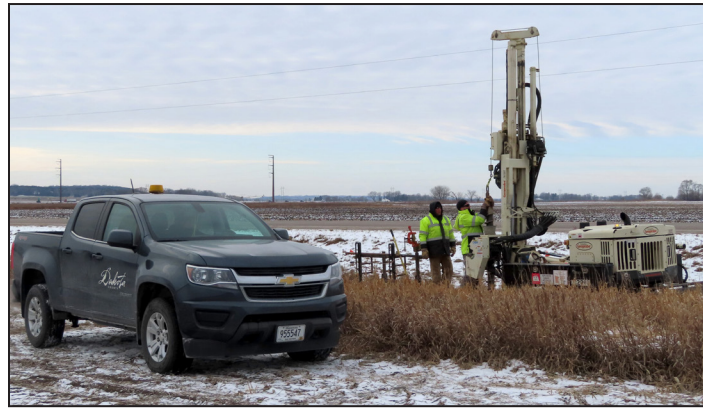
A Midwestern Drilling crew used a hollow-stem auger to drill one of Dakota County’s ACRE monitoring wells in Hampton Township. Dakota County will use results from the rural monitoring well network and its private well sampling programs to track trends in groundwater and drinking water chemicals to evaluate progress of the ACRE program. Photo Credit: Dakota County staff
