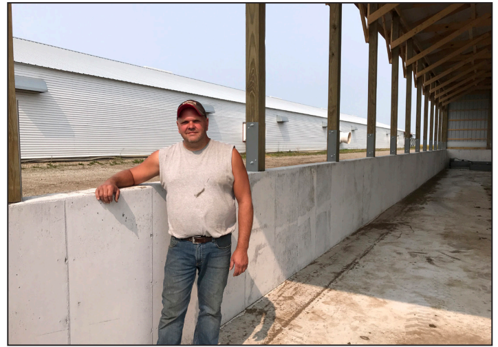
Left, from left: Shirley and Kevin Klaphake told Mike Hemmann, a Stearns County-based NRCS civil engineering technician, and Stearns County SWCD Project Management Supervisor Nathan Hylla how a newly constructed, roofed stacking slab built to store 12 months of poultry litter fit into their operation. Right: Meyer, seen here shortly after a 40-by-100-foot covered stacking slab was constructed near the poultry barn on his Lake Henry Township farm, said having 12 months' storage made it possible to incorporate that nitrogen source in the fall.
