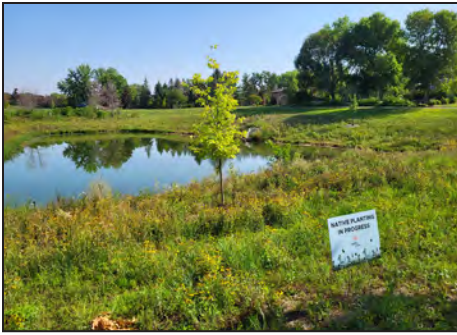
Left: The city of Apple Valley and the VRWJPO used a BWSR Watershed-Based Implementation Funding grant to retrofit a stormwater pond in Erickson Park in 2021. The project provides additional water-quality treatment and infiltration, resulting in better management and treatment of low flows, a reduction in phosphorus delivery to Farquar Lake, and better access for maintenance. Middle: The segment of the Vermillion River within Rambling River Park in Farmington is impaired for turbidity, dissolved oxygen and aquatic life. An Aug. 23 tour stop highlighted a trout stream restoration, which involved planting native seeds, constructing bioengineering practices and excavating soil to better connect the Vermillion River to its floodplain. Right: The city of Lakeville and the VRWJPO were among the partners involved in the King Park stormwater reuse system project, one of eight stops on the summer tour. A pump system reuses and moves water from the stormwater ponds to irrigate the park's baseball fields.
