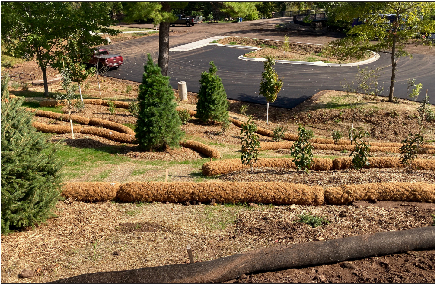
Bioswales, biofiltration basins, rock-armored culverts and native plantings are part of the BWSR Clean Water Fund-backed stormwater management work, installed in conjunction with other park improvements, that will benefit temperature-impaired Miller Creek.
