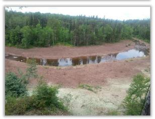
*Pictured, top: Construction of the new bank. Pictured, bottom: Floodplain bench installed at the bank stabilization site on the Knife River.*
