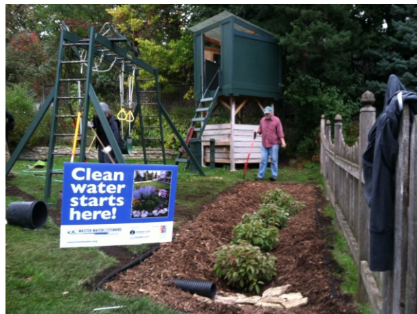
A resident installs a rain garden as part of a local conservation project.
