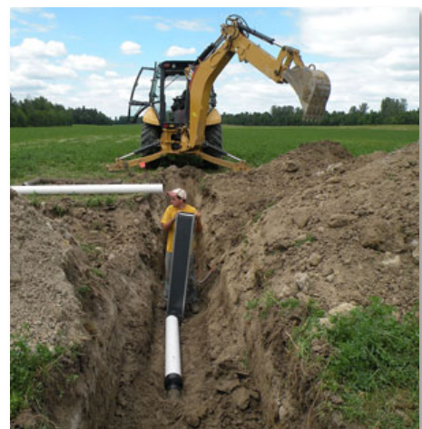
Workers installing an outlet for a water and sediment control basin.
