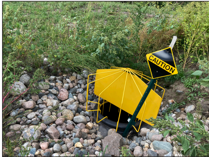
Above: A gully once cut into Joe Ste. Marie's Terrebonne Township field and sent topsoil down a cliff to a Clearwater River tributary. A diversion and intake now channel the runoff, slow it down and allow sediment and the pollutants it carries to settle out. A pipe carries the water, which is filtered before it reaches the river. Below: Sun filters through clouds over a Red Lake County field.
