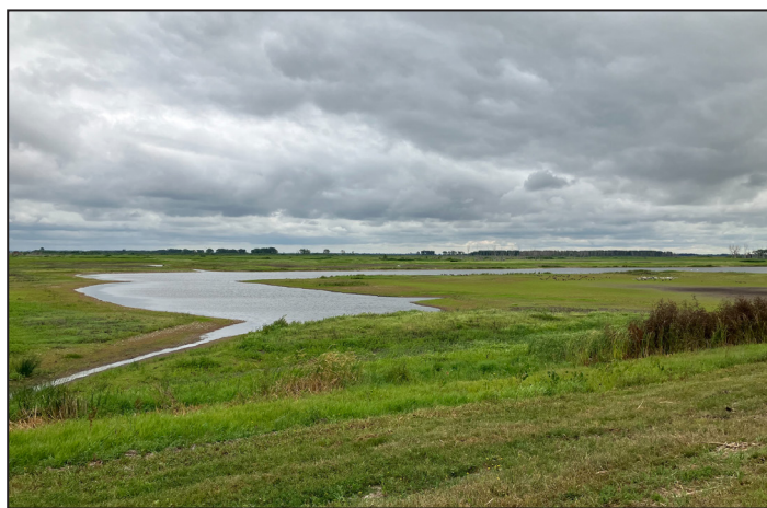
The Agassiz Valley Water Resources Management Project was developed under a mediation agreement between the state of Minnesota and the Red River Watershed Management Board. It was designed for flood control and environmental enhancements, and spans about 2,600 acres in Marshall and Polk counties.
