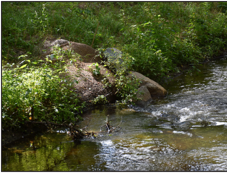
Left: The first stage of the CCWD’s Clean Water Fund-supported work on Sand Creek in Coon Rapids focused on Lower Sand Creek corridor restoration. Construction included five backwater pools, and six rock cross vanes designed to control the grade and direct stream flow. The project incorporated toe wood protection, resloping, and vegetated rock riprap streambank stabilization techniques. Middle: CCWD Water Quality Coordinator Justine Dauphinais walked along Sand Creek in fall 2019. Right: Most of Sand Creek functions as a ditch; only the downstream 2.2 miles function as a stream. Photo Credits: Ann Wessel, BWSR
