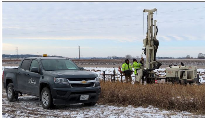
A Midwestern Drilling crew used a hollow-stem auger to drill one of Dakota County’s ACRE monitoring wells in Hampton Township. Dakota County will use results from the rural monitoring well network and its private well sampling programs to track trends in groundwater and drinking water chemicals to evaluate progress of the ACRE program. Photo Credit: Dakota County staff
