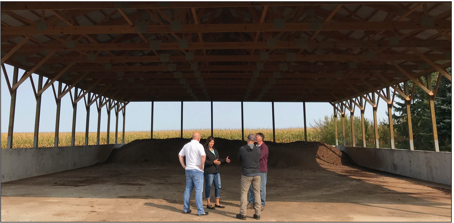
Shirley and Kevin Klaphake, in back, told NRCS civil engineering technician Mike Hemmann, in white, and Stearns County SWCD Project Management Supervisor Nathan Hylla how a newly constructed, roofed stacking slab built to store 12 months of poultry litter fit into their operation.
