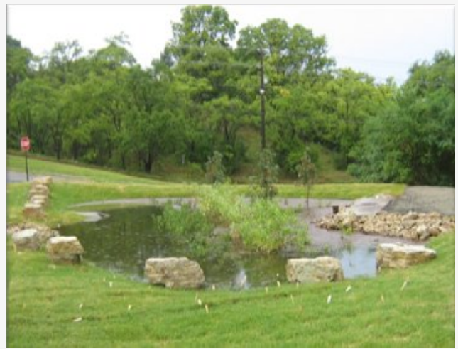
After: S. St. Paul Stormwater Retrofits at Wakota Ice Arena
