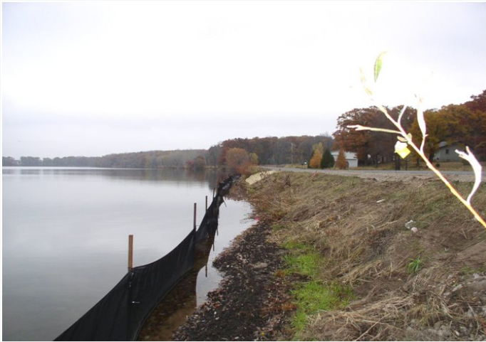
Lake Freemont Shoreline Restoration Project, Livonia Township
