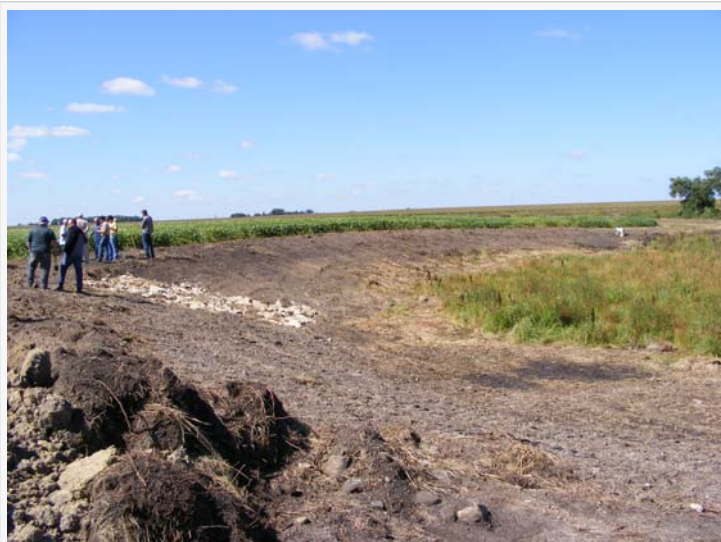
Looking downstream across the length of the bioreactor
