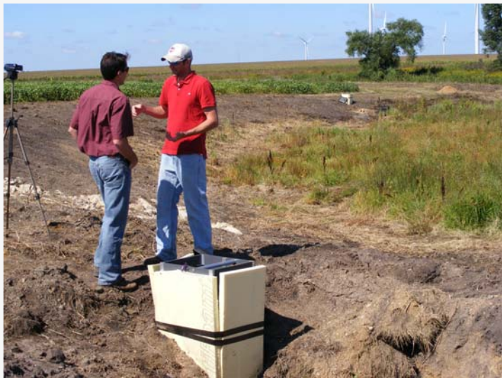
A lowflow bioreactor inlet control structure
