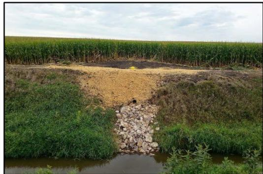
Ditch Side Inlet Structure - Drop Inlet
