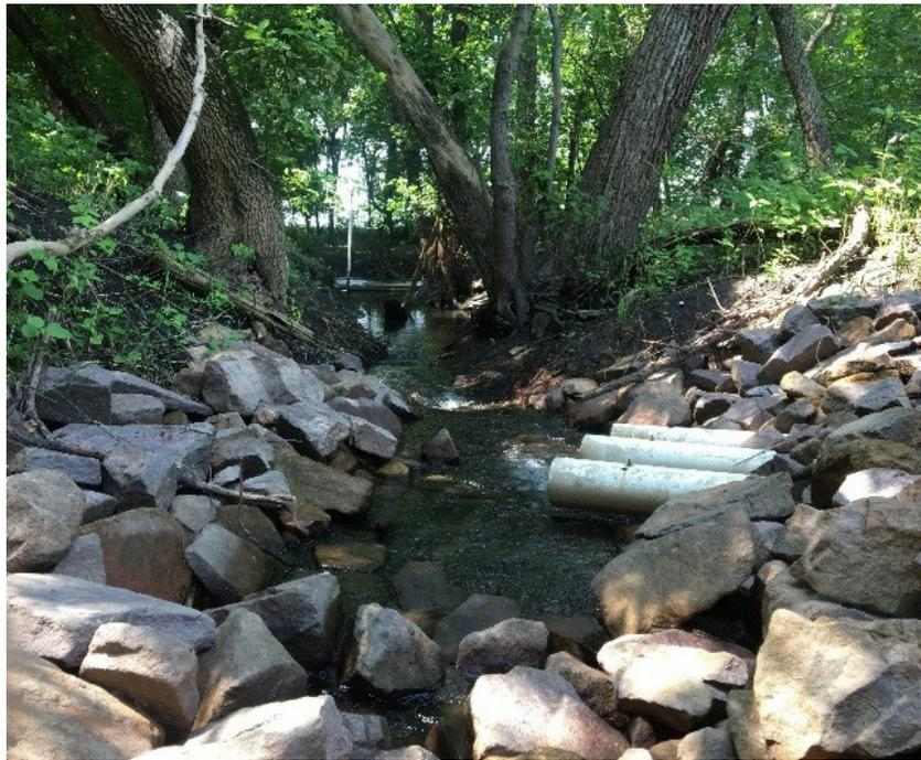
*Outlet pipes for a treatment wetland plus a bioreactor meant to reduce nitrate-nitrogen are elements of a "treatment train," which strings together a series of practices to maximize pollution reduction. It replaced the saturated buffer originally proposed.*
