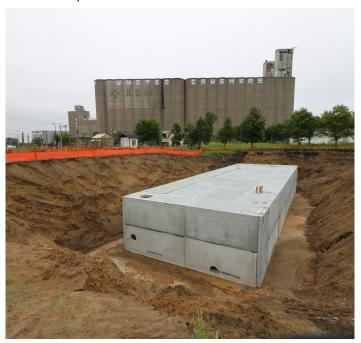
The storage tank beneath the main basin can hold up to 206,575 gallons of treated runooff.
