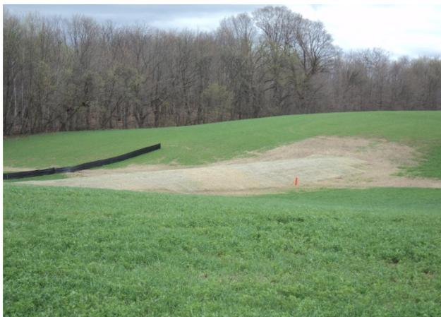
*Gully Project Site C before and after installation of a Water and Sediment Control Basin to stabilize gully erosion.*
