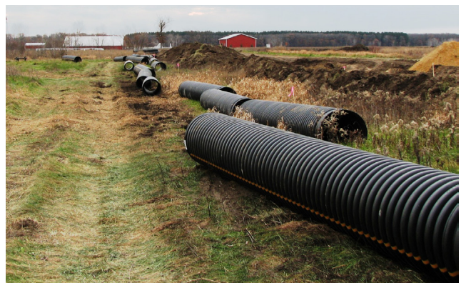
Figure 3.69 Installation of Diversion Pipe
