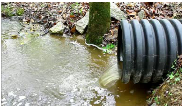
Figure 3.65 Storm Sewer Outlet
