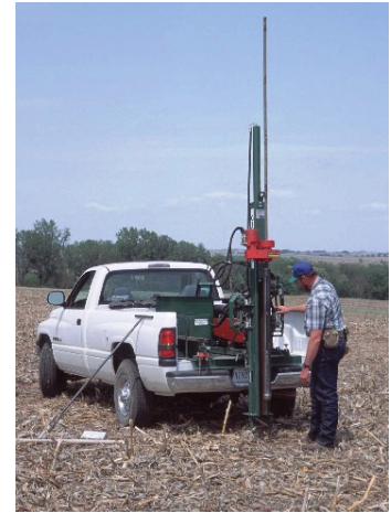
Figure 3.18 Soils Assessment with Drill Rig
