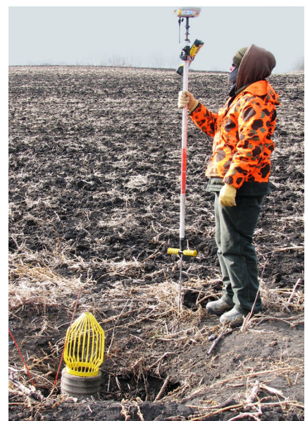
Figure 3.59 Surveying Underground Drain Tile
