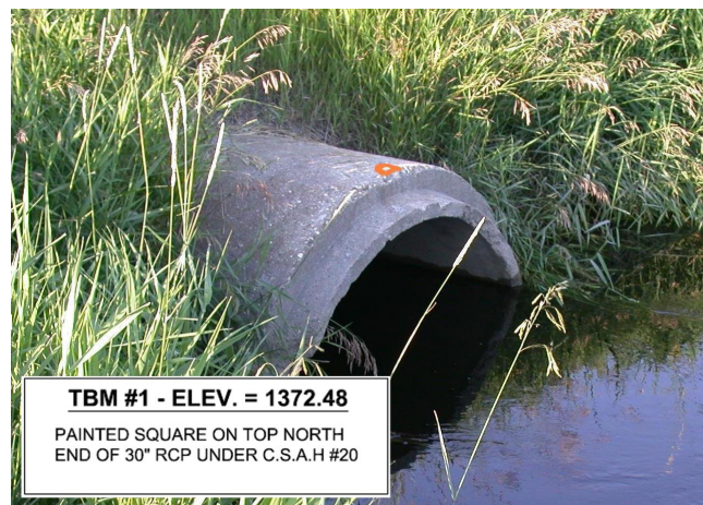
Figure 3.52 RCP Culvert used as a TBM
