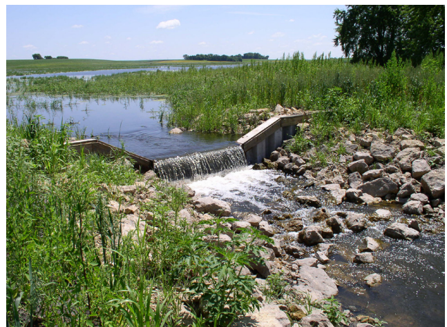
Figure 3.21 Outlet Structure on Restored Wetland
