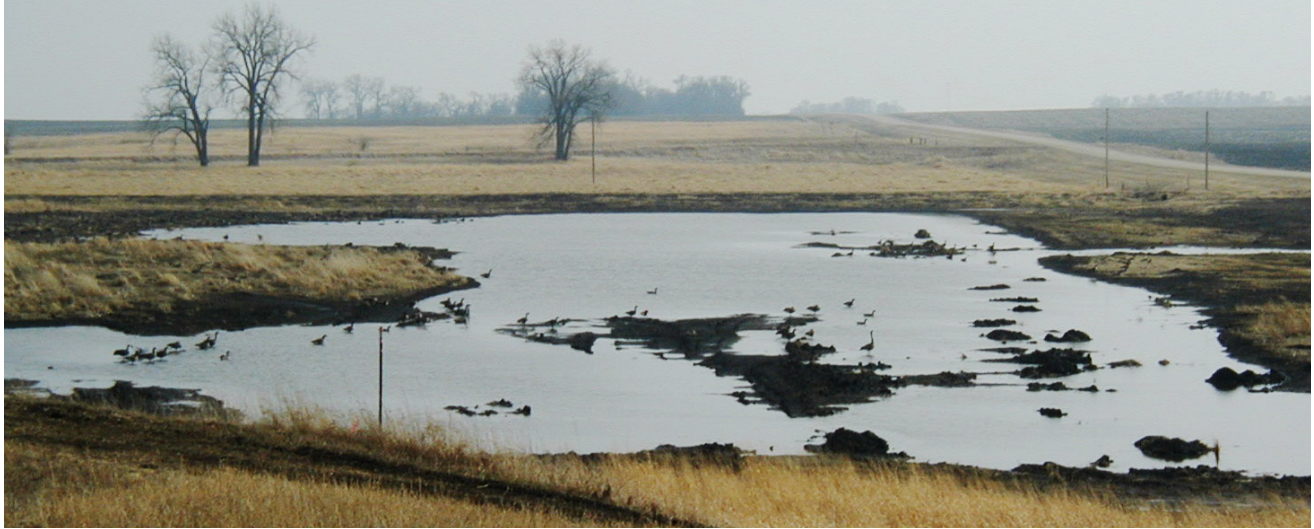
Figure 3.19 Recently Constructed Wetland Excavation
