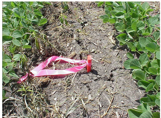
Figure 3.55 Wood Hub used as Construction TBM
