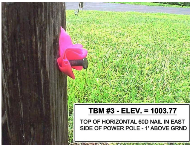
Figure 3.53 Spike in Power Pole used a TBM
