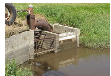
Figure 3.62 Drainage Lift or Pump Station
