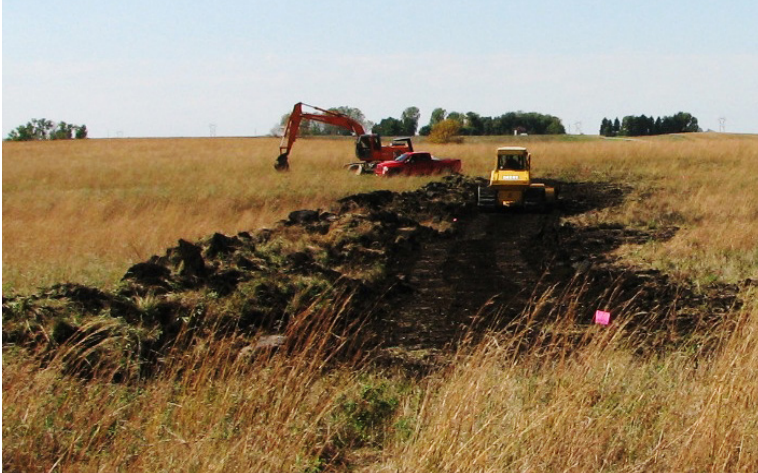
Figure 3.14 Topsoil Stripping
