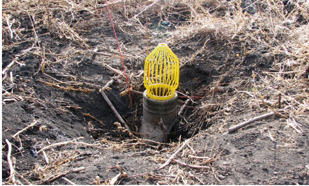
Figure 3.36 Subsurface Drainage Tile Intake
