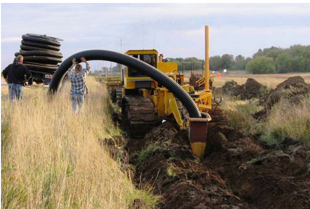
Figure 3.26 Installation of Drainage Tile
