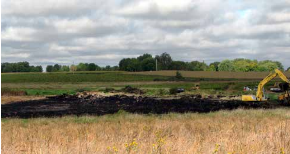
Figure 4.6.4 Sediment Being Removed from Wetland Edge
