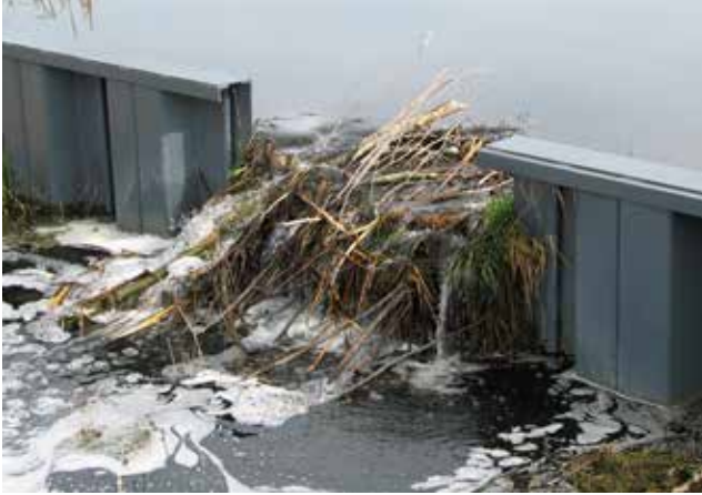
Figure 4.4.14 Plugged Outlet Caused by Beaver
