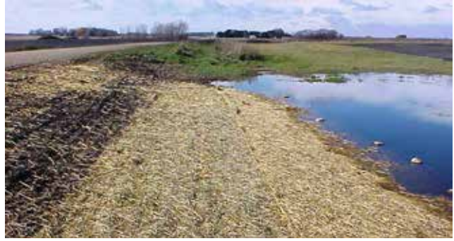
Figure 4.7.6 Earthen Berm Against Road Slope
