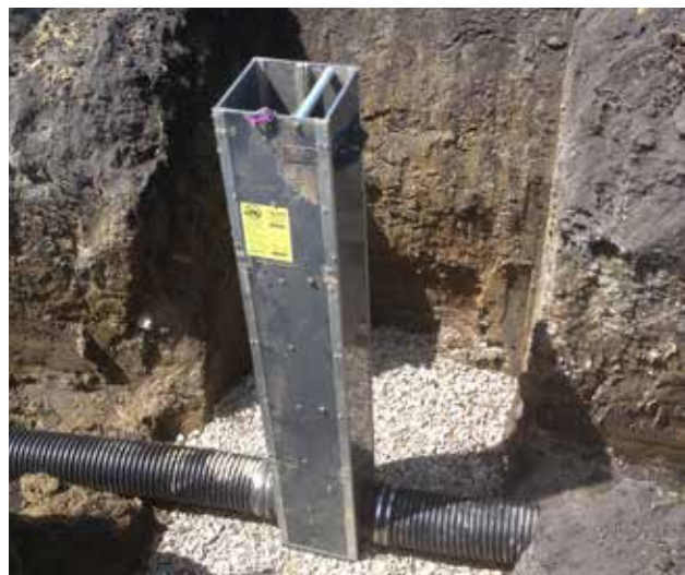
Figure 4.4.27 In-Line Water Level Control Structure
