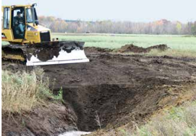
Figure 4.3.5 Construction of a Ditch Plug
