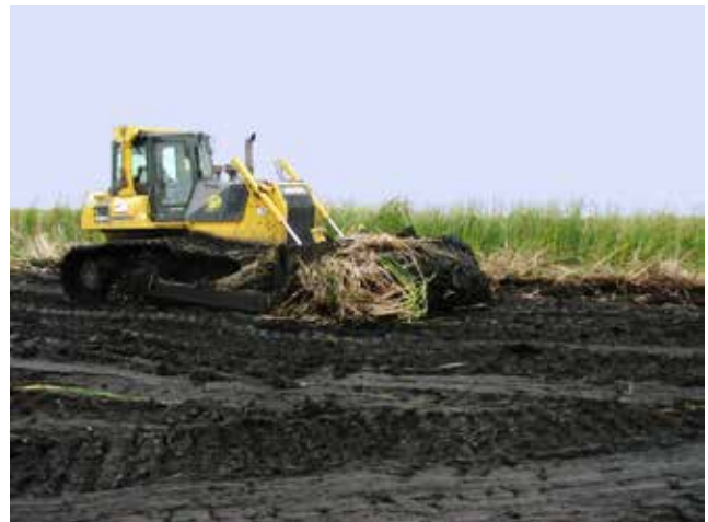
Figure 4.6.2 Excavation to Remove Undesired Cattail
