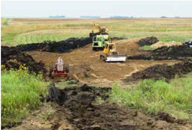
Figure 4.9.1 Construction Site Excavation
