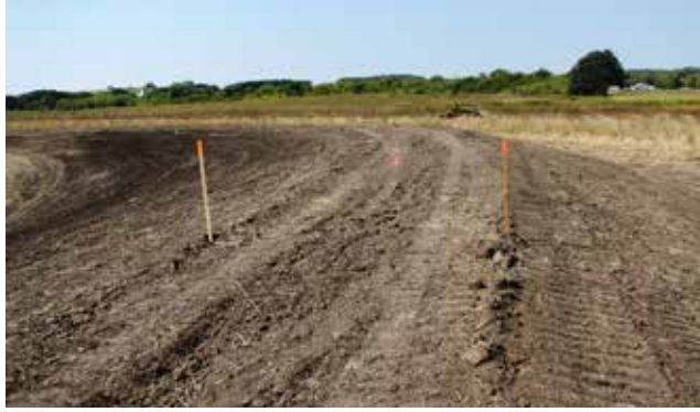
Figure 4.5.4 Curvilinear Embankment Alignment with Relatively Flat Side Slopes
