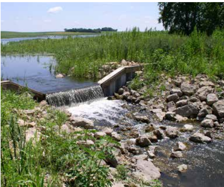
Figure 4.4.1 Wetland Outlet Structure
