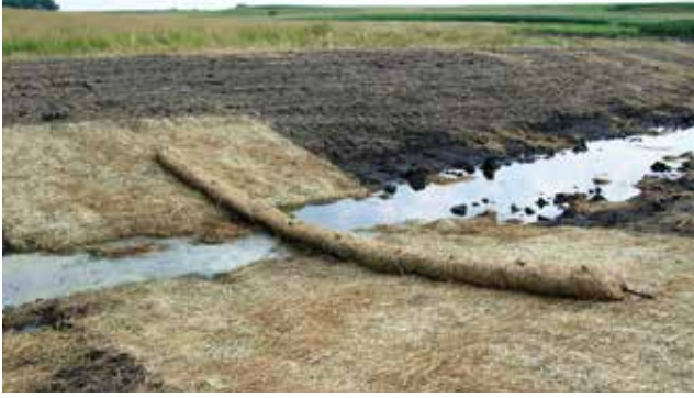
Figure 4.9.3 Sediment and Erosion Control Practice
