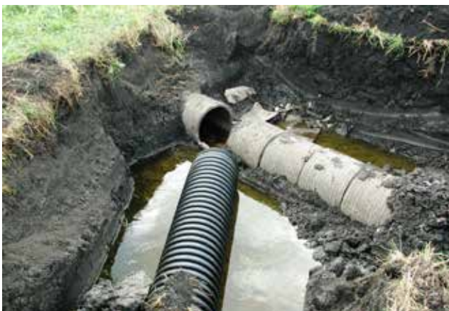
Figure 4.3.4 Subsurface Drainage Tile
