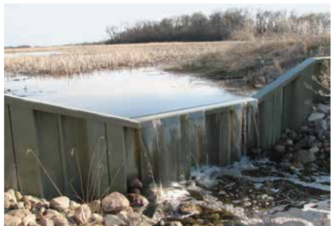
Figure 4.4.28 Vertical Fish Barrier
