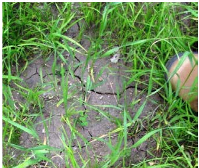
Figure 4.5.8 Embankment Soils Fracturing
