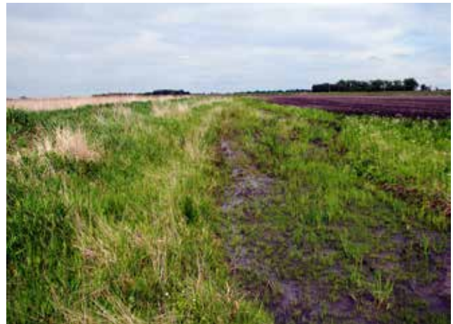
Figure 4.5.11 Wetness on Downstream Side of Embankment Due to Seepage
