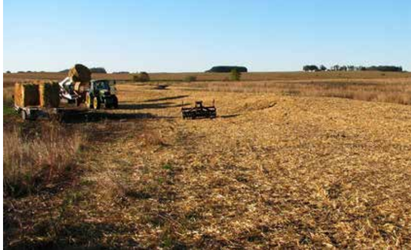
Figure 4.5.24 Placing Mulch on a Constructed Embankment
