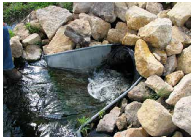
Figure 4.4.4 Flow at Entrance to Horizontal Culvert
