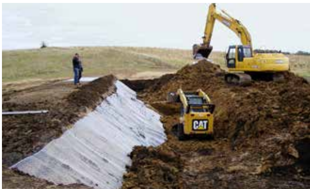
Figure 4.5.33 Installation of a Rodent Fence in Embankment
