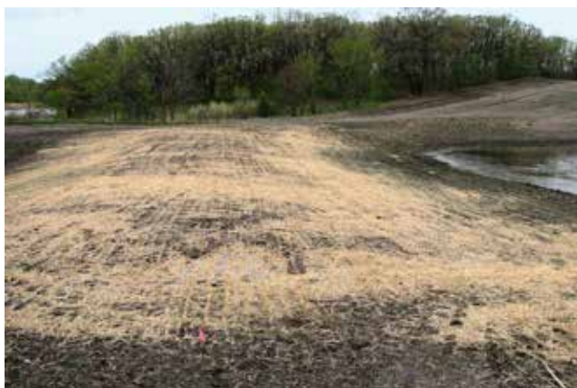
Figure 4.5.20 Embankment with a Gradual Front Slope
