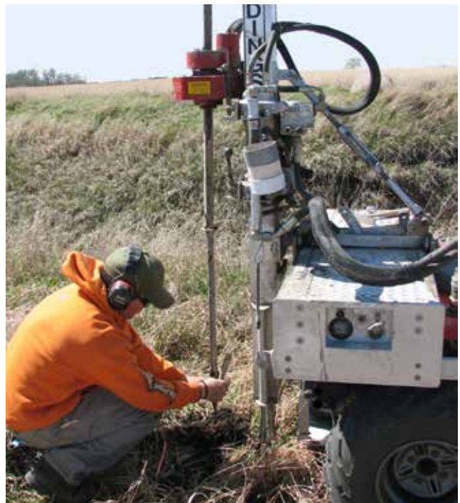
Figure 4.5.14 Soils Foundation Investigation
