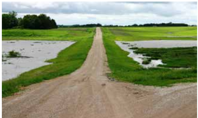
Figure 4.7.8 Improved Road Bed – Post Construction
