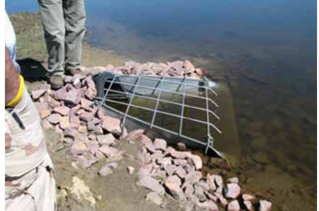
Figure 4.4.17 Trash Guard on Culvert End
