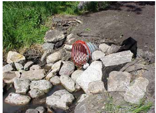
Figure 4.4.18 Hinged Rodent Guard on Pipe Outlet
