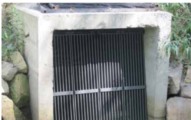
Figure 4.4.31 Swinging Fingers on Box Culvert Outlet
