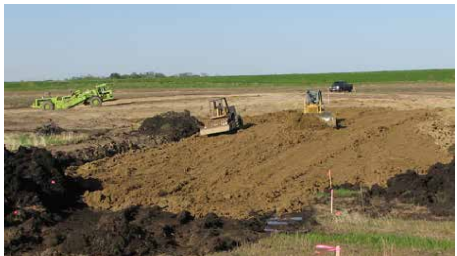
Figure 4.10.11 Earthen Embankment Under Construction
