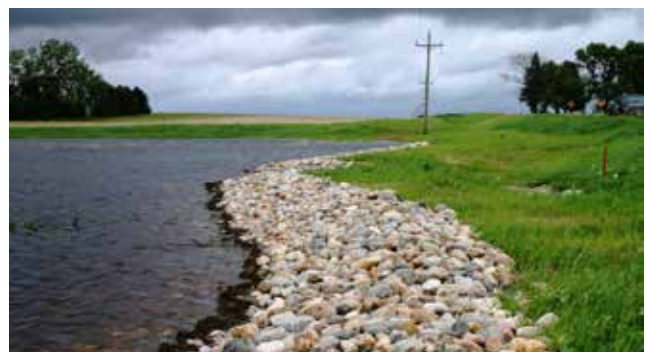
Figure 4.5.27 Embankment Slope Protected with Riprap
