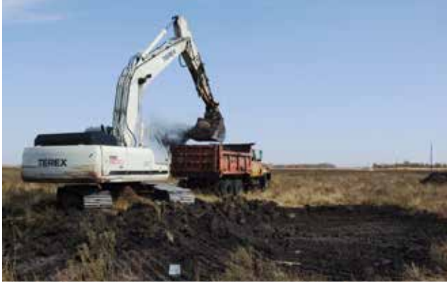
Figure 4.2 Excavation Work on a Construction Site
