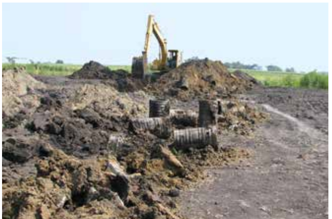
Figure 4.3.7 Construction of a Tile Block
