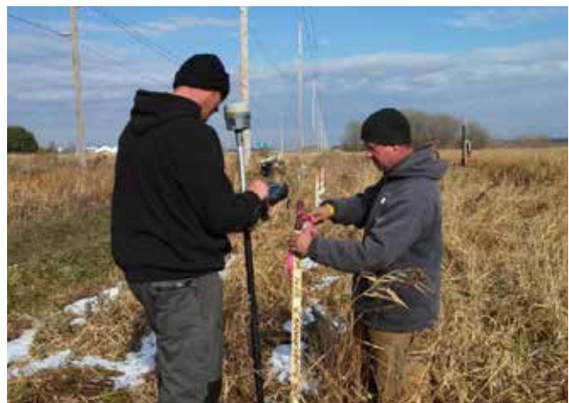
Figure 4.10.4 Layout and Staking Process
