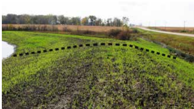
Figure 4.5.19 Cross Section of Embankment Showing Slightly Crowned Top
