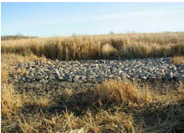
Figure 4.4.2 Rock Weir Structure
