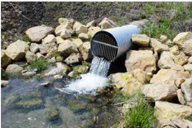
Figure 4.3.8 A Constructed Tile Outlet
