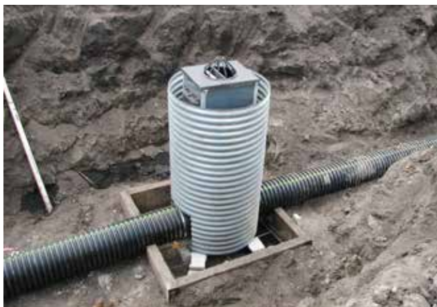
Figure 4.4.12 Preparing for a Concrete Footing on an In-Line Water Level Control Structure
