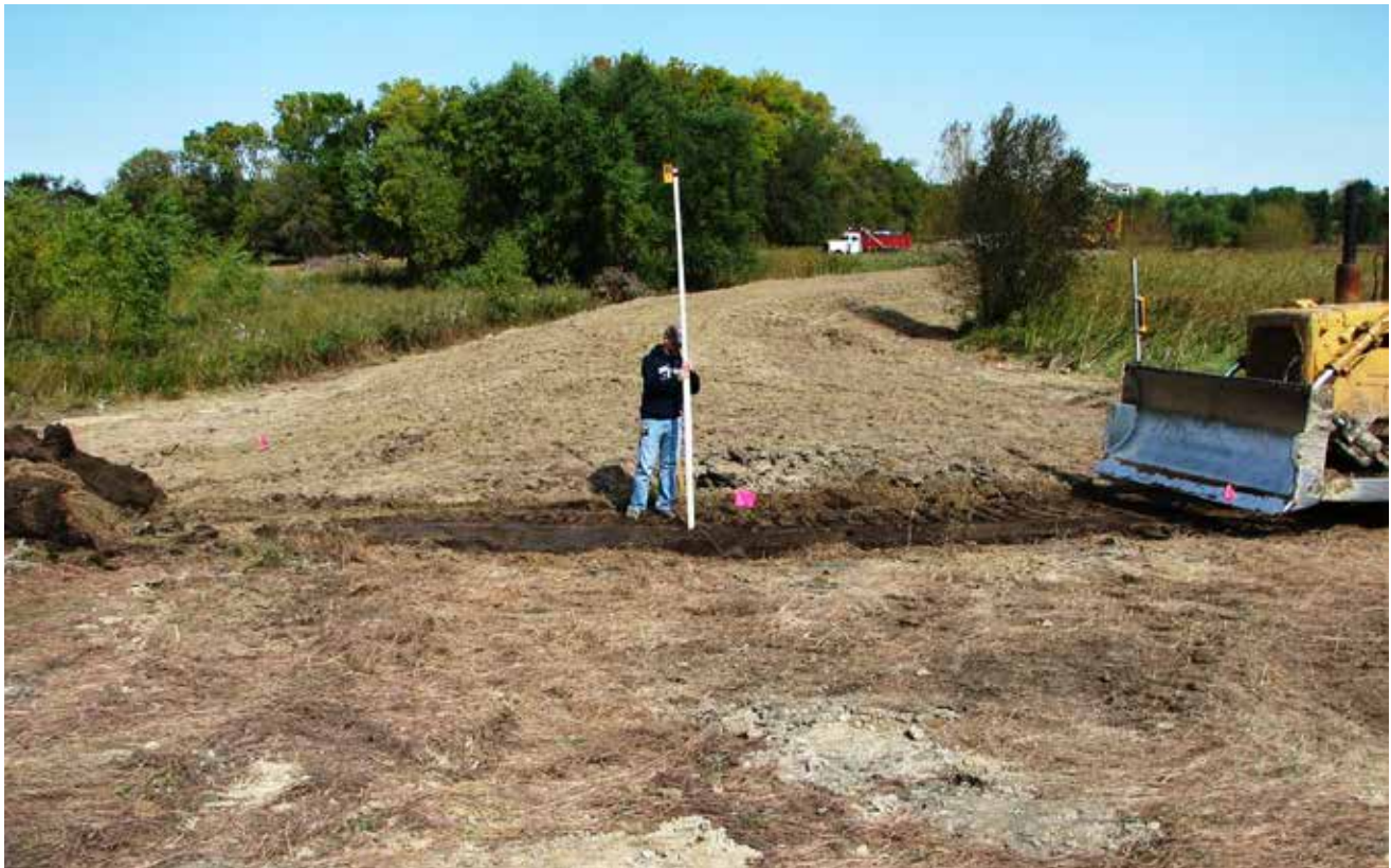
Figure 4.10.15 Checking Construction Work
