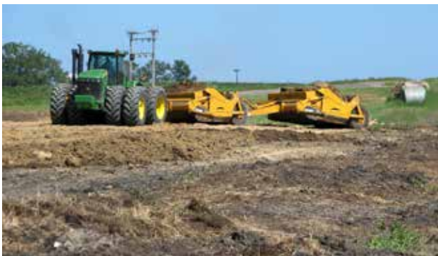
Figure 4.5.23 Embankment Compaction with Loaded Tandem Scrapers
