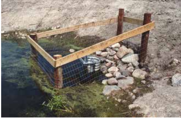
Figure 4.4.22 Fence Barrier Around Drop Inlet Structure
