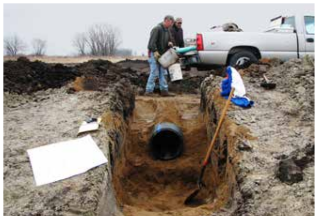
Figure 4.4.13 Installing Sand Drainage Diaphragm and Filter at Outlet End of Pipe Structure
