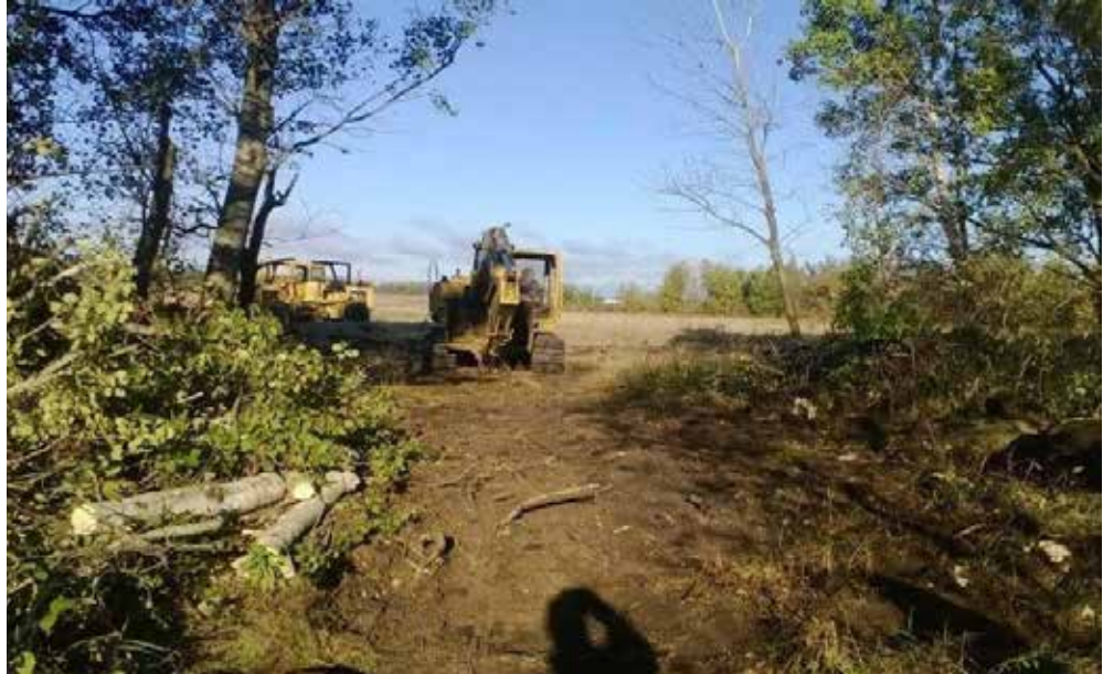
Figure 4.10.9 Clearing and Grubbing of Planned Embankment Area
