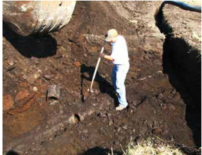
Figure 4.10.12 Construction of Tile Block/Removal
