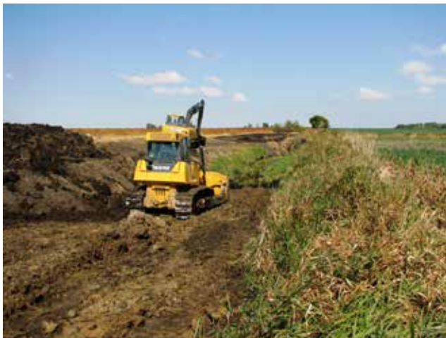
Figure 4.3.9 Improving a Ditch Bank to Restore a Wetland
