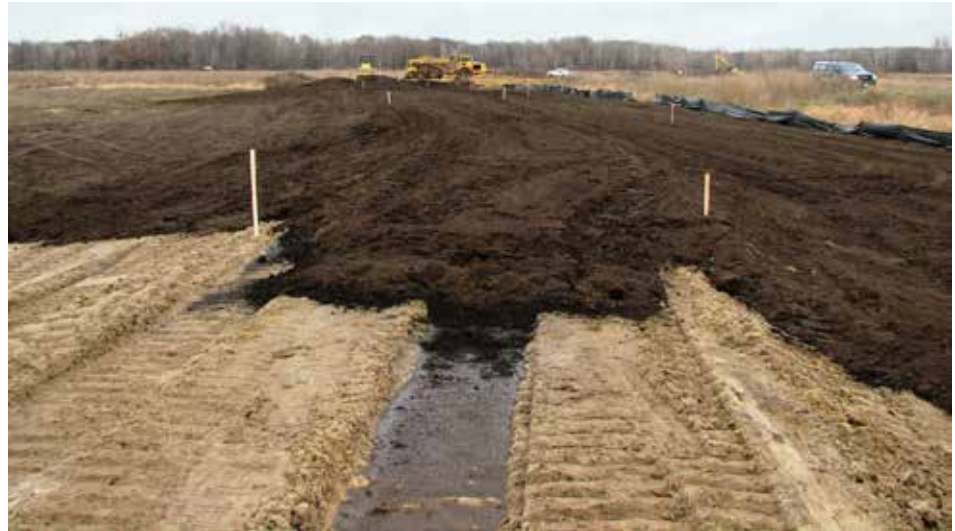
Figure 4.10.15 Placing Topsoil on Constructed Embankment
