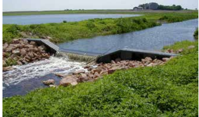
Figure 4.4.6 Steel Sheet Pile Weir Structure
