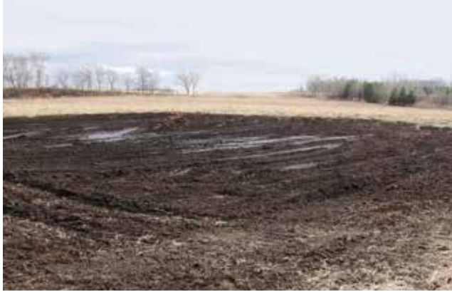
Figure 4.6.10 Finished Grade of Wetland Scrape
