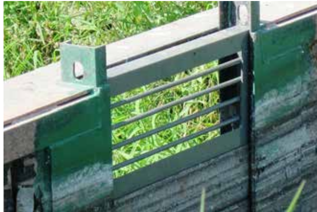
Figure 4.4.30 Vertical Screen Barrier
