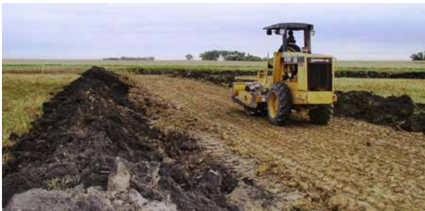
Figure 4.5.21 Embankment Compaction with Sheepsfoot Roller
