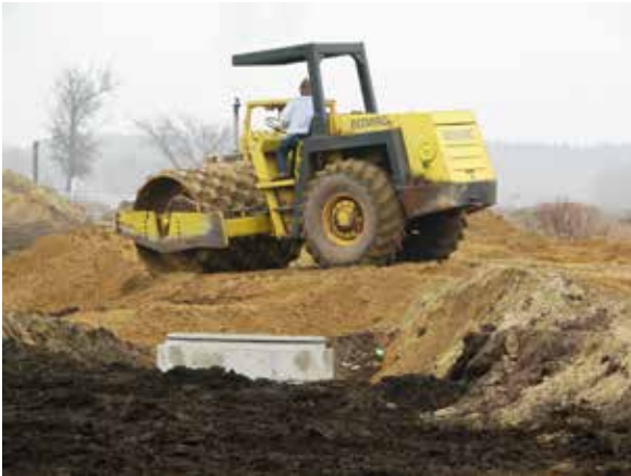
Figure 4.10.1 Project Site Construction
