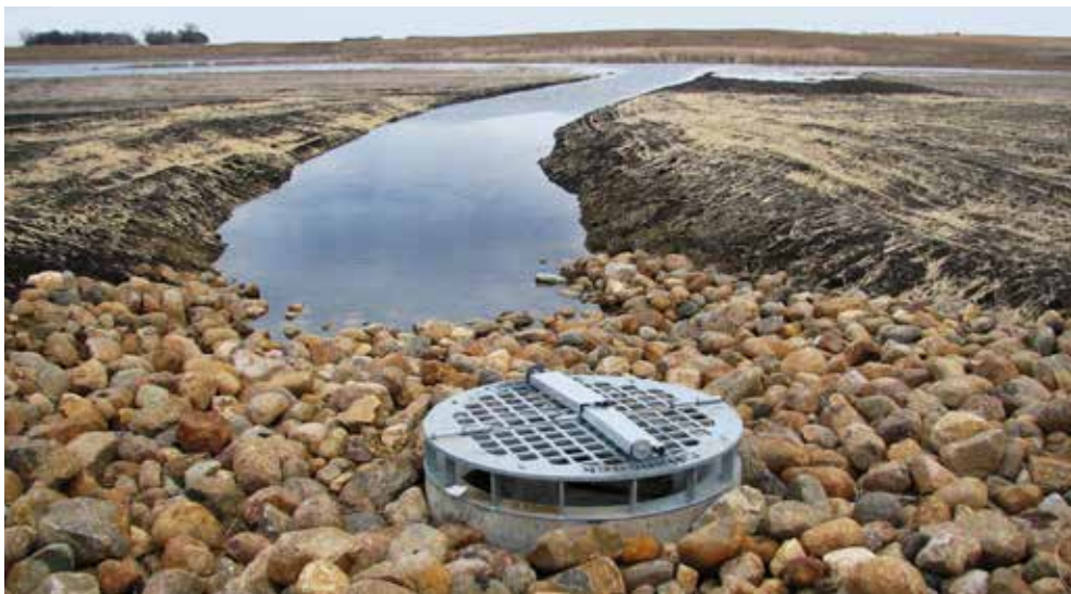
Figure 4.4.23b Rock Filter Enclosure of Riser
