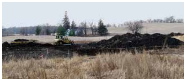
Figure 4.6.6 Excavated Sediment Being Placed as Loose Fill on Adjoining Property
