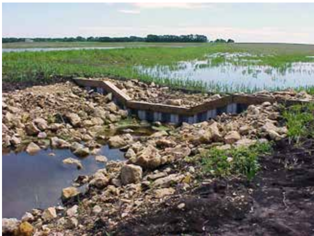
Figure 4.10.14 Rock Riprap at Wetland Outlet
