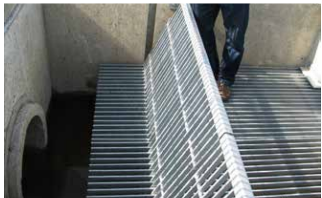
Figure 4.4.32 Horizontal Screens with Vertical Swinging Fingers
