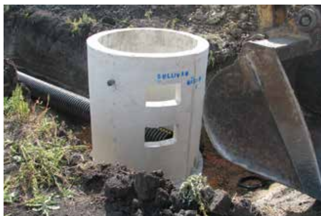
Figure 4.4.11 Installation of a Reinforced Concrete Catch Basin Outlet Structure
