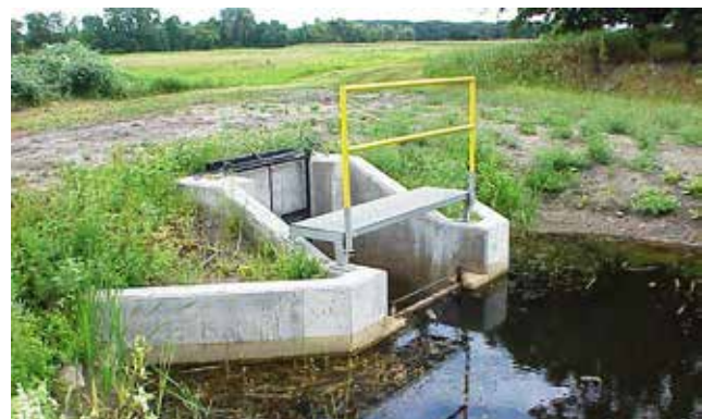
Figure 4.4.25 Concrete Drop Structure with Stoplog Bay
