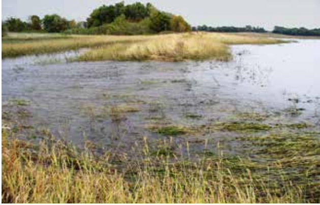
Figure 4.4.8a Vegetated Spillway After Large Runoff Event
