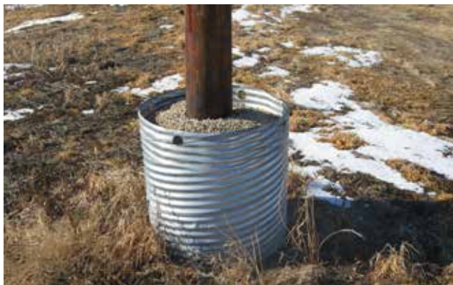
Figure 4.7.11 Sleeve Protection of Utility Poleland
