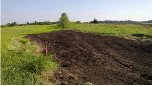
Figure 4.7.3 Fill Placed and Graded to Protect an Adjacent Property
