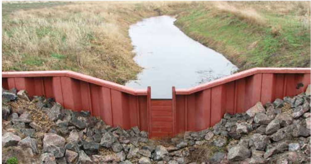
Figure 4.4.26 Steel Sheet Pile Weir with Stoplog Bay for Managing Water Levels
