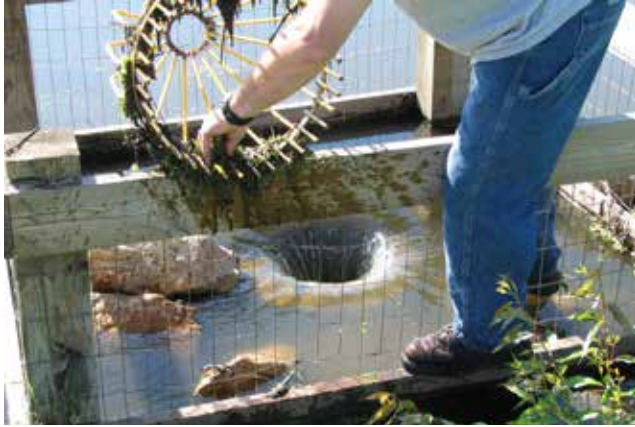
Figure 4.4.16 Removing Debris from Plugged Trash Guard
