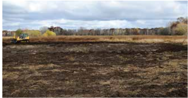
Figure 4.6.9 Topsoiling of Excavated Scrape Area
