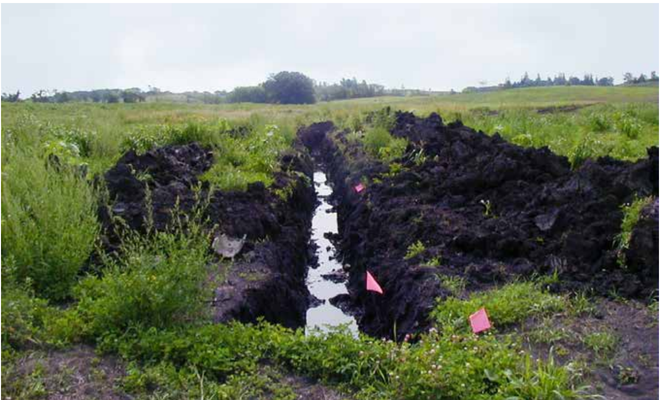
Figure 4.10.7 Tile Block Location Marked with Flags
