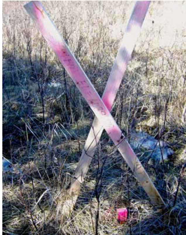
Figure 4.10.5 Temporary Construction Hub
