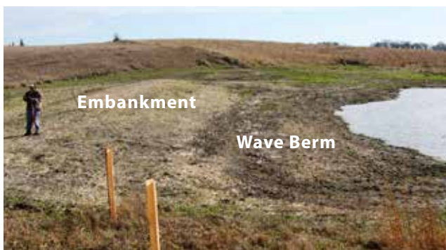
Figure 4.5.26 Embankment Protected with Wave Berm
