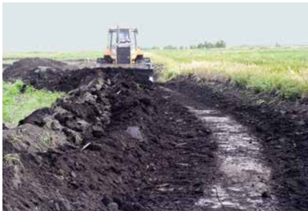
Figure 4.5.13 Stripping Topsoil at Embankment Site
