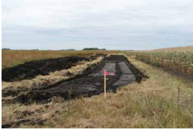
Figure 4.10.10 Stripping Topsoil Under Planned Embankment
