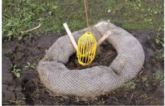
Figure 4.10.8 Sediment Protection of Functioning Tile Inlet
