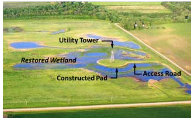
Figure 4.7.12 Earthen Pad and Access Road to Utility Tower
