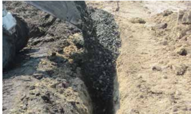
Figure 4.5.31 Construction of Aggregate Barrier
