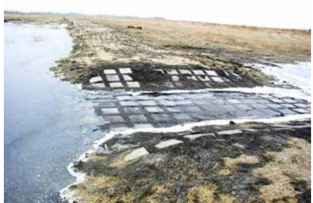
Figure 4.4.9 Cable Concrete Armored Spillway
