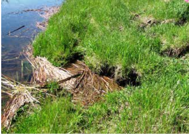
Figure 4.5.28 Muskrat Damage to Embankment
