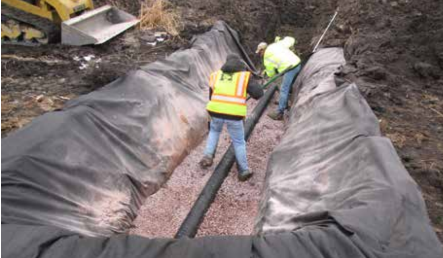
Figure 4.4.24a Trickle Drain with Aggregate Drain Filter
