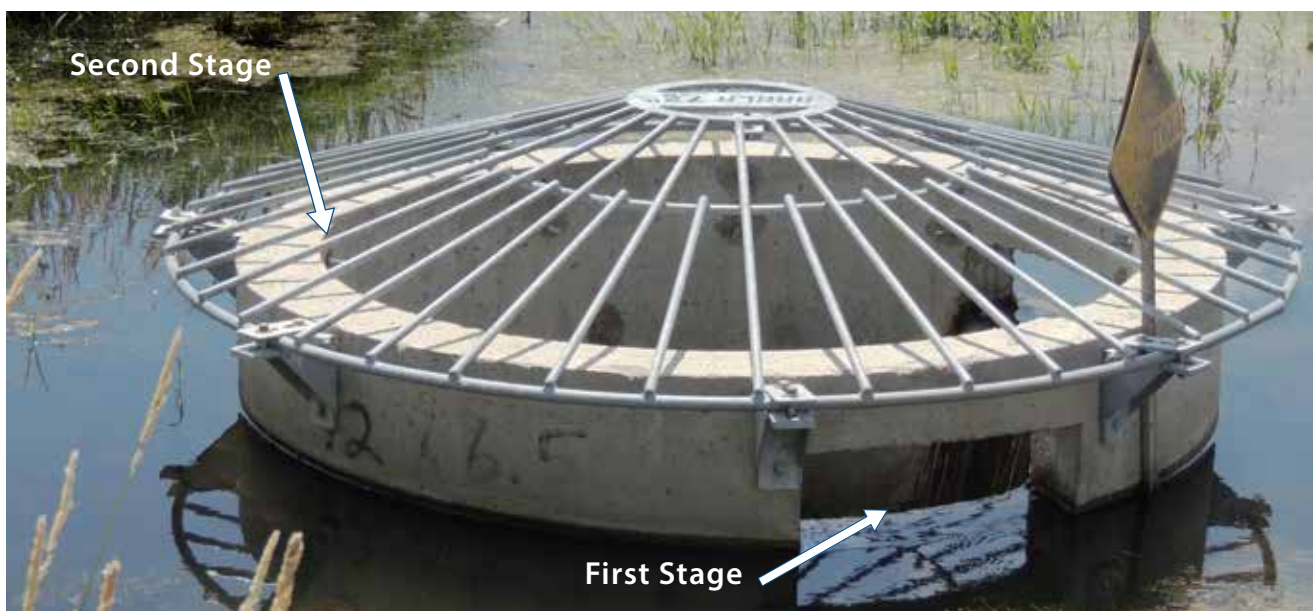
Figure 4.4.10 Multi-Staged Concrete Drop Inlet Structure- Note Orifice Opening at Water Surface
