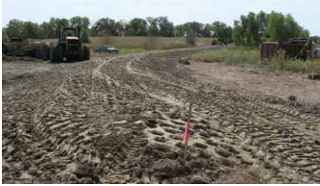
Figure 4.5.2 Wetland Embankment Under Construction
