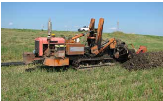
Figure 4.3.1 Installation of Drainage Tile
