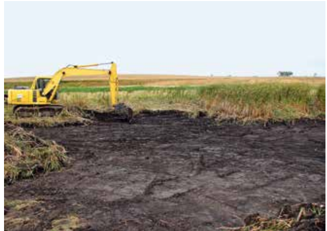
Figure 4.6.3 Sediment Removal from Partially Drained Wetland
