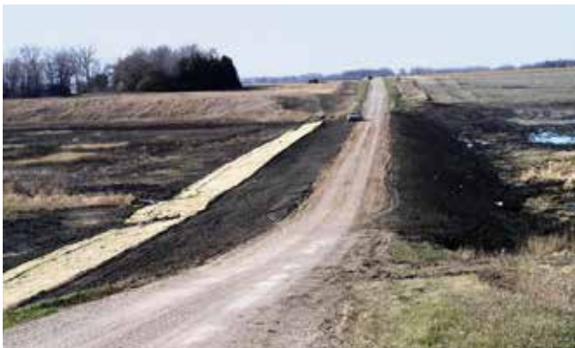
Figure 4.7.7 Road Bed and R-O-W Being Improved as Part of a Wetland Restoration
