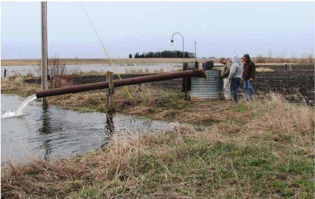
Figure 4.3.10 A Relocated Tile Drainage Lift Station Discharging into a Restored Wetland
