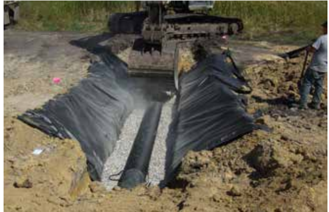
Figure 4.4.3 Construction of a Trickle Drain
