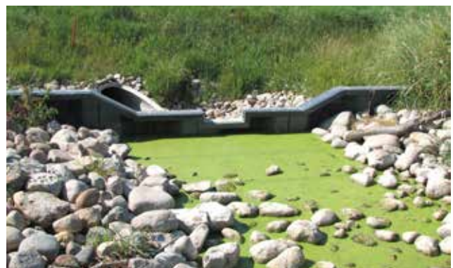
Figure 4.4.7 2-Stage Weir
