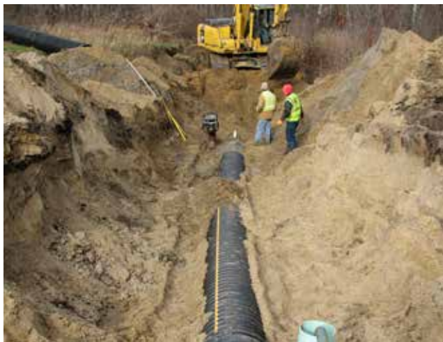
Figure 4.10.13 Compacting Around Outlet Pipe
