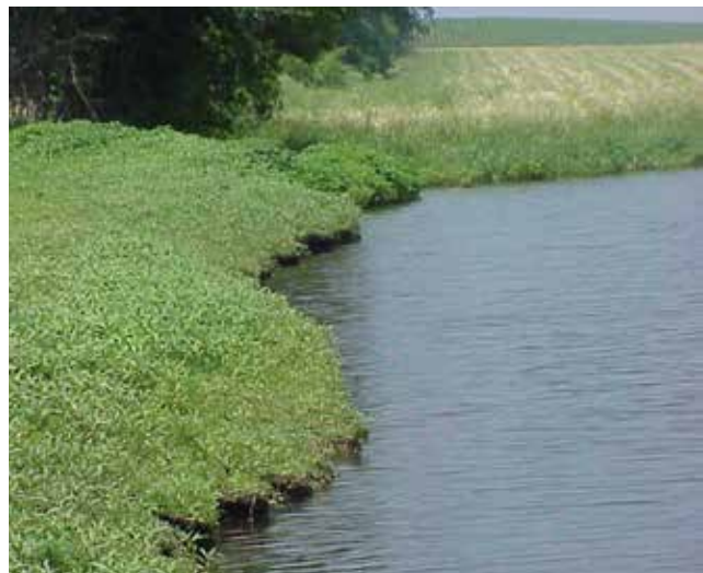
Figure 4.5.25 Embankment Damage from Wave Action
