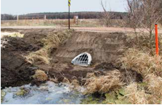
Figure 4.7.9 New Culvert Thru Road as Wetland Outlet
