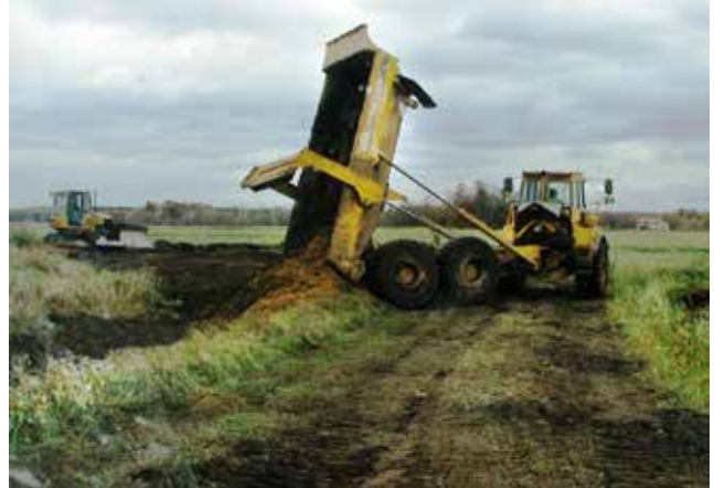
Figure 4.3.6 A Drainage Ditch Being Filled In
