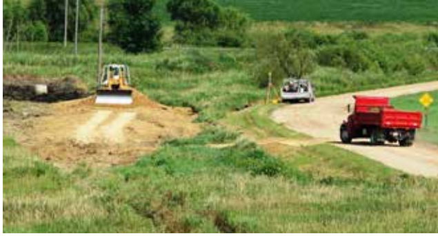
Figure 4.7.5 Embankment Being Constructed to Protect Adjacent Road
