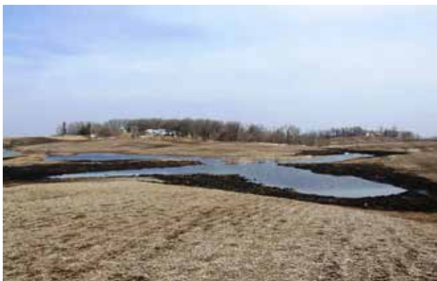
Figure 4.6.5 Wetland Scrape with Irregular Edges
