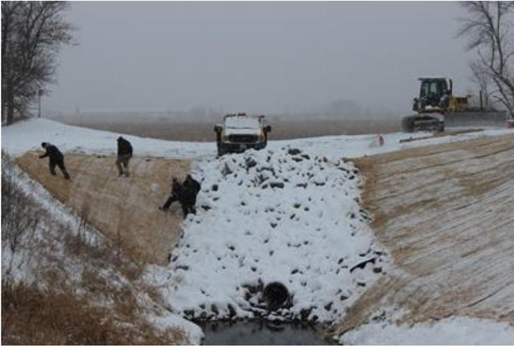
*Erosion & sediment control applied during snowstorm as project nears completion.*
