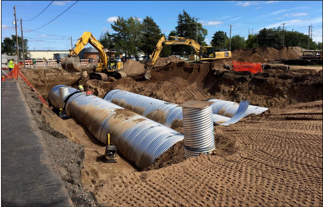
Workers installed an underground stormwater treatment system in northeast St. Cloud, where untreated stormwater previously drained into the Mississippi River. A $705,000 Clean Water Fund grant from the Minnesota Board of Water and Soil Resources helped pay for the system. Below: A sump manhole, showed during cleaning, acts as a mini treatment system. Photo Credits: Benton SWCD
