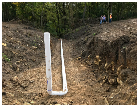
Above: Mark and Judy Diercks walked along a 440-foot-long berm at the edge of their Belvidere Township field while a contractor built the dam designed to stop gully erosion. Below, from left: Beau Kennedy of the Goodhue Soil & Water Conservation District discussed the project with the Diercks. A retention basin was designed to hold water for up to 12 hours on the field, and then meter it out slowly through a 6-inch pipe. Lake Pepin will benefit from upland conservation practices funded in part by a Clean Water Fund grant from the Minnesota Board of Water and Soil Resources.
