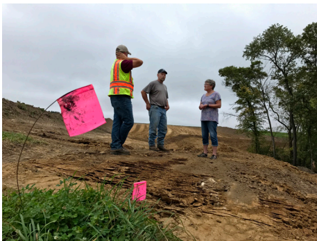
Above: Mark and Judy Diercks walked along a 440-foot-long berm at the edge of their Belvidere Township field while a contractor built the dam designed to stop gully erosion. Below, from left: Beau Kennedy of the Goodhue Soil & Water Conservation District discussed the project with the Diercks. A retention basin was designed to hold water for up to 12 hours on the field, and then meter it out slowly through a 6-inch pipe. Lake Pepin will benefit from upland conservation practices funded in part by a Clean Water Fund grant from the Minnesota Board of Water and Soil Resources.
