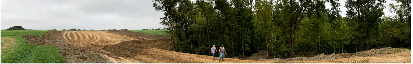
Above: Mark and Judy Diercks walked along a 440-foot-long berm at the edge of their Belvidere Township field while a contractor built the dam designed to stop gully erosion. Below, from left: Beau Kennedy of the Goodhue Soil & Water Conservation District discussed the project with the Diercks. A retention basin was designed to hold water for up to 12 hours on the field, and then meter it out slowly through a 6-inch pipe. Lake Pepin will benefit from upland conservation practices funded in part by a Clean Water Fund grant from the Minnesota Board of Water and Soil Resources.
