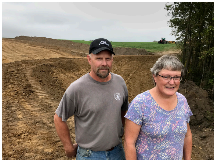
Mark and Judy Diercks stood at the edge of their bluff-top field where dams installed as part of Goodhue SWCD’s effort to curb upland gully erosion will cut the amount of sediment entering trout streams in the Mississippi River/Lake Pepin watershed.
