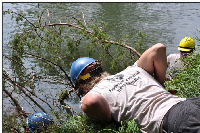
Teamwork was especially important for the Conservation Corps Minnesota & Iowa crew working along a section of Riceford Creek with steeper banks. Brennen Reyscak, 24, of Ankeny, Iowa, handed down tools to fellow crew members on Aug. 15, 2018, in Houston County.
