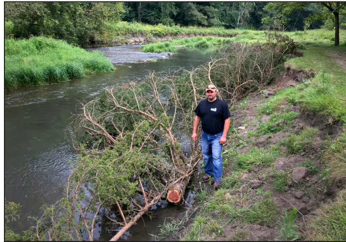
Dustin Looman, assistant district manager for Conservation Corps Minnesota & Iowa's South Region, explained cedar revetment work on Riceford Creek in Houston County.
