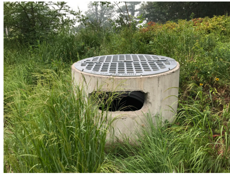
A two-stage retention basin and iron-enhanced sand filter slow and treat runoff from a 30-acre drainage area in Deerwood, removing about 90% of the phosphorus. At the Summer Place on Serpent Lake, heavy rains had flooded some — but not all — of the 13 cabins. Getting all 13 property owners to agree to the project generated conflict and negotiation because those unaffected by flooding didn't want to give up land.
