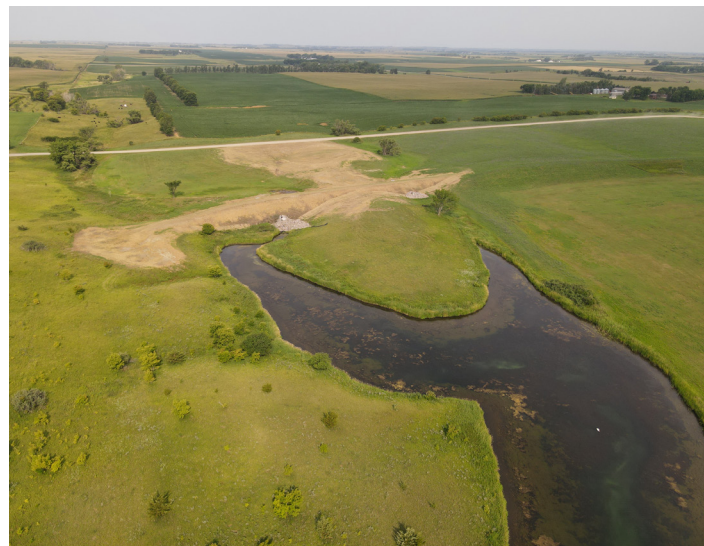
Two grade stabilization structures share a berm on the northwest side of Del Clark Lake. The two structures, plus a roadside retention embankment near the south area of the lake, are estimated to capture a combined 667 tons of sediment each year.
