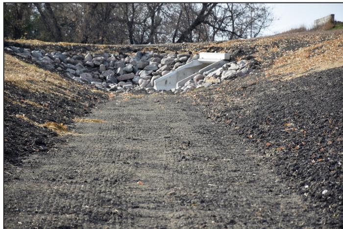
*Side-water inlets, top, are part of the BDSWD’s multipurpose drainage management work on Traverse County Ditch 35 supported by a Clean Water Fund grant from BWSR. The project has water storage, water quantity and water quality benefits. Work finished in fall 2022. Above: In Redpath Township, Traverse County Ditch 35 outlets into Twelvemile Creek through a culvert. The ditch, seen here in October 2022, would usually contain water that time of year.*
