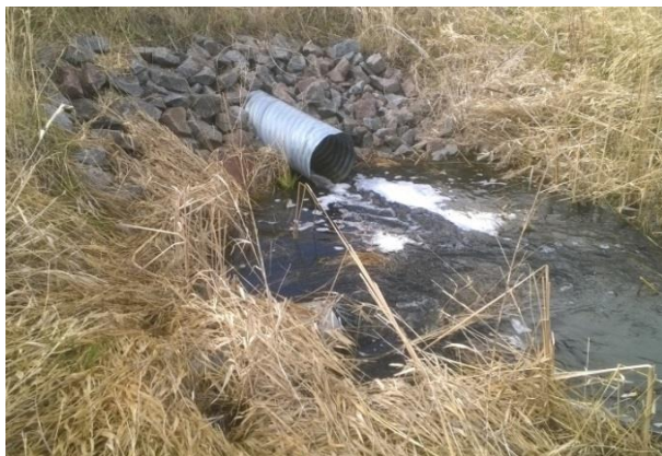
Figure 1. Upstream Drainage Tile Outletting into Restored Wetland
