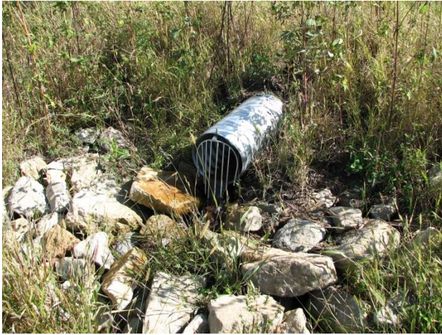
Figure 6. Riprap Protection at Tile Outlet
