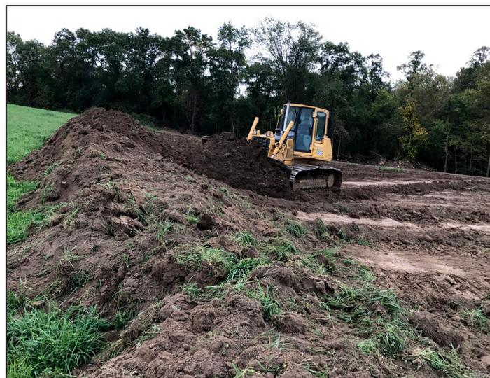
Jesse Hadler of Hadlers Dozin of Lake City scraped away the topsoil to expose the clay that would build the berms of a dam being constructed on Mark and Judy Diercks' Belvidere Township field.
