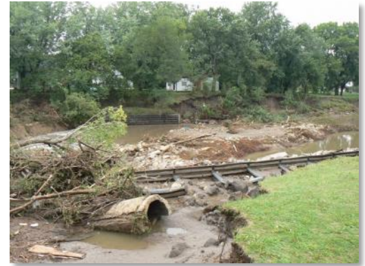
Flood damage in southeastern Minnesota
