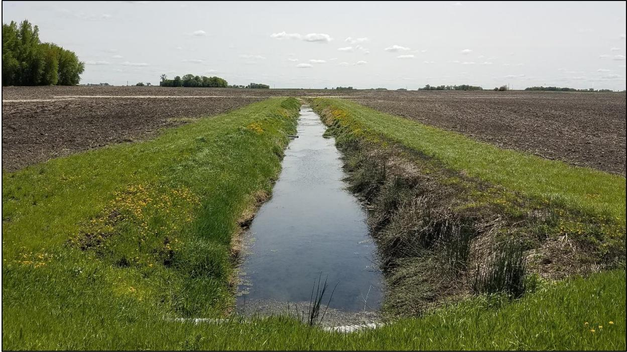
Example Chapter 103E Drainage Ditch with Buffer Strips
