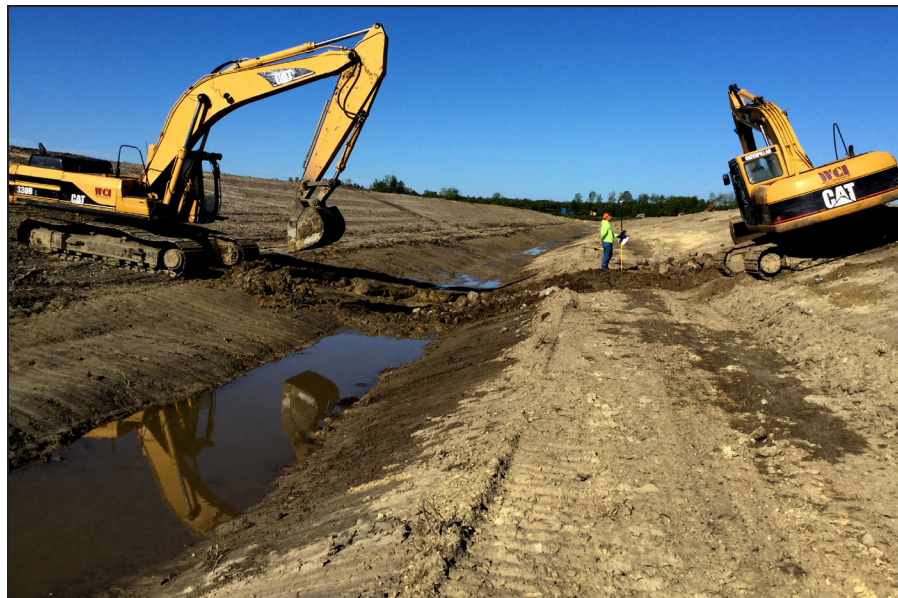
Wyatt Erickson, a Lake of the Woods Public Works Department engineering technician, helps to set elevations where the contractor is installing a rock riffle. Photo Credit: Lake of the Woods SWCD
