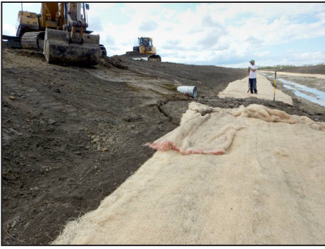
Left: A Wright Construction employee stands on the bench where a side-water inlet is being installed. Judicial Ditch 28 channel stabilization work was completed this summer. Middle: Direct construction costs totaled about $250,000. Among the other project costs are engineering, surveying and inspection work; administration; project development; education and outreach, which is planned for this spring. Right: “Our goal is to have more stable ditch banks,” Trask said. Photo Credits: Lake of the Woods SWCD
