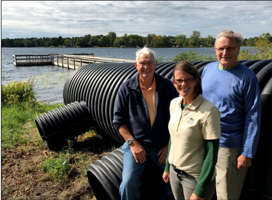
Crow Wing Soil & Water Conservation District Manager Melissa Barrick visited the site of a stormwater treatment project in Crosby on Sept. 18 with Serpent Lake Association members Clark Marshall, left, and Arlen Bowen.
