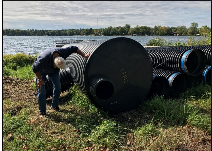
Above: Arlen Bowen of the Serpent Lake Association inspects a sediment trap Sept. 18. It will be installed as part of a stormwater treatment project in Crosby, replacing a pipe that released untreated stormwater directly into Serpent Lake.
