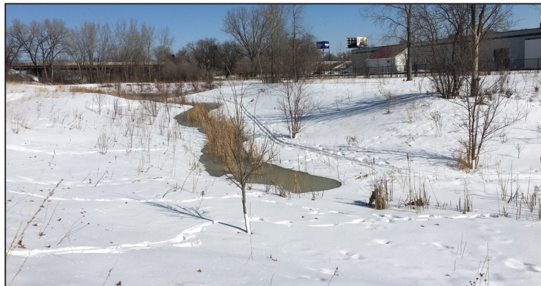
The project, which finished in February 2020, required pumping water from a stormwater sewer interceptor on one side of the railroad tracks under the active rail line to the stream on the other side. Photo Credit: City of St. Paul
