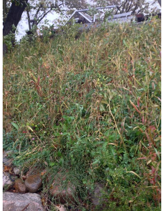
Steep bank stabilized with flowers, grasses and erosion control blanket
