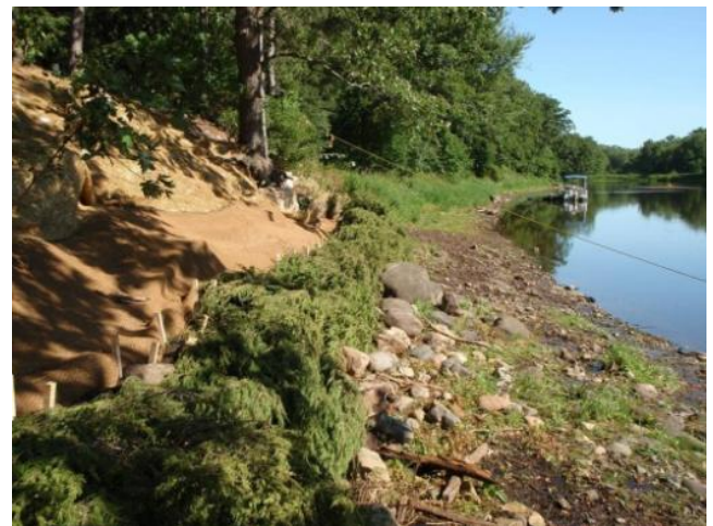
Bank stabilization with cedar revetments and erosion control
